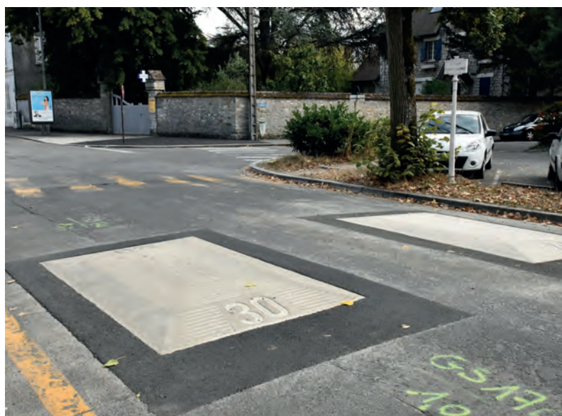
→ Installation de coussins berlinois boulevard Churchill
