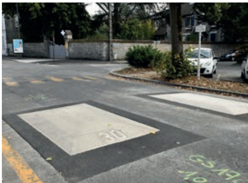
→ Installation de coussins berlinois boulevard Churchill
